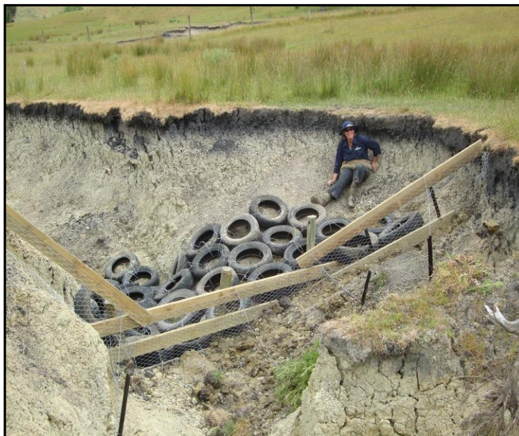
Netting debris dam : note the back fill upstream of the structure, standards to tie the structure back, wings above flood level, weir board horizontal and tyres downstream.
